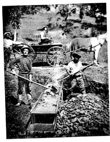
Miners shoveled gravel into a narrow box called a *sluice*. The water running through washed away the lighter particles, and the gold remained.
